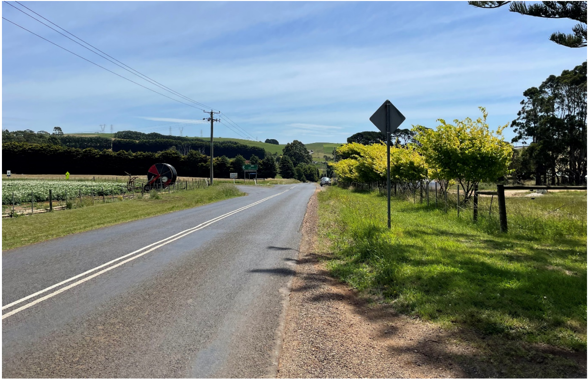
Figure 3 – Existing Pine Road junction.
