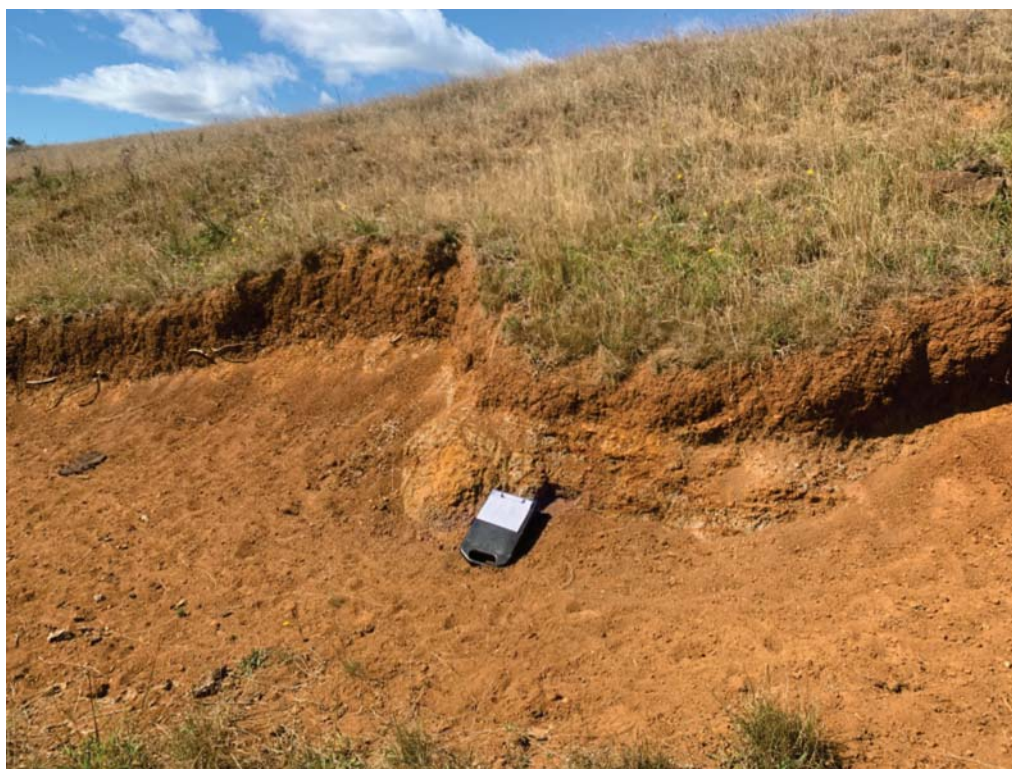
PLATE 6 - Looking south at the cut batter of the existing access road to Lot 2 and Lot 3. Soil profile consists of shallow residual soil overlying extremely/highly weathered rock.
