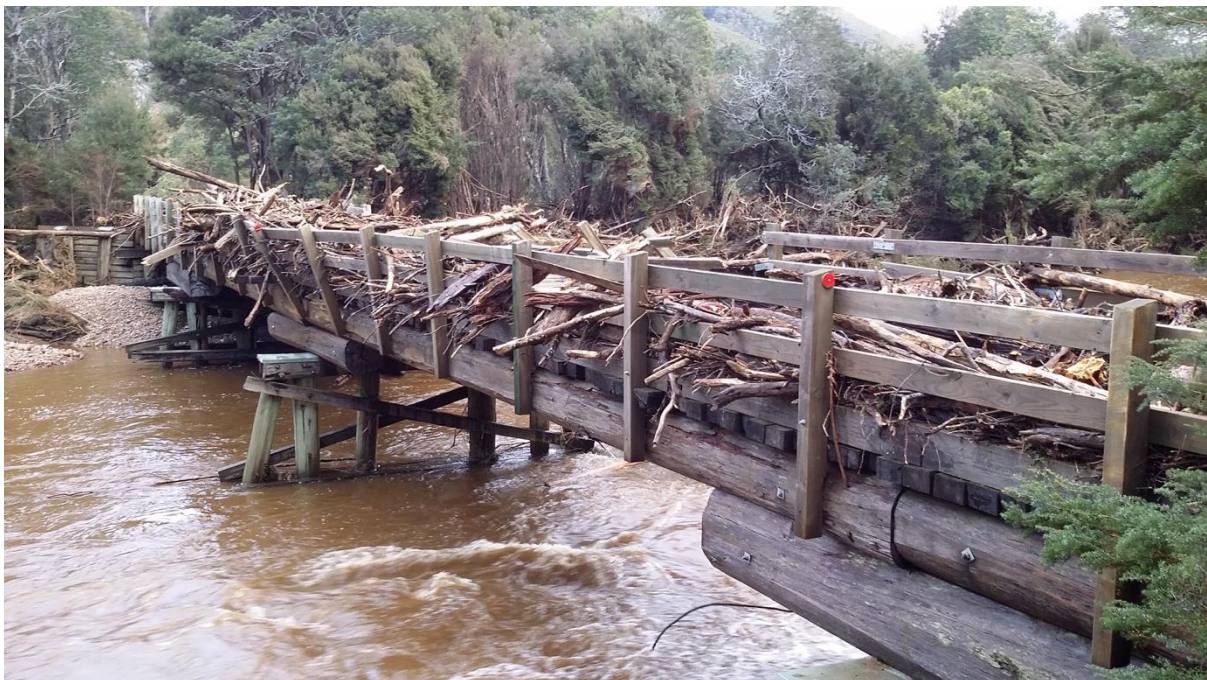
Figure 1. Flood damage to Council bridge at Taylors Flat (2016)
