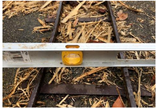
Photo 2 Track out of level by 16mm of west curve.
