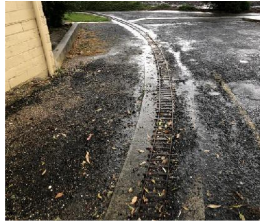
Photo 8 Closer sleeper spacing to stiffen the track
