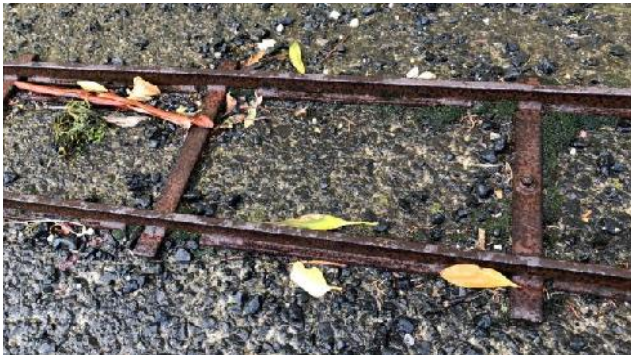
Photo 11 Track with stiffener plate below rail
