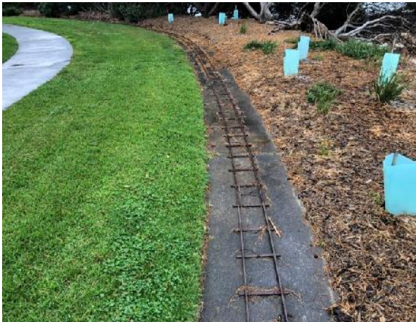
Photo 9 Area where occasional sleepers need replacing
