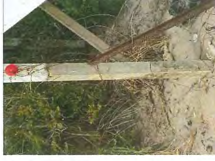
(The white paint marks the sand level prior to November 2007)
