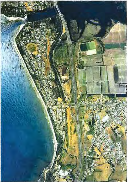
Figure 2. 2005 Aerial photograph of Turners Beach shows the wave refraction at the shoreline in proximity to the Boys Road – Esplanade intersection.
